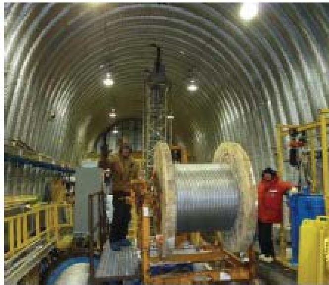
Spooling on the new 4,200 m cable
