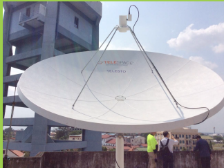
GOES, COMS, MTSAT, FY2 GVAR/LRIT/HRIT/SVISSR MODEL: 3.7m
