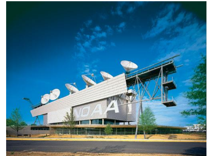
NOAA Satellite Operations Facility (NSOF)
