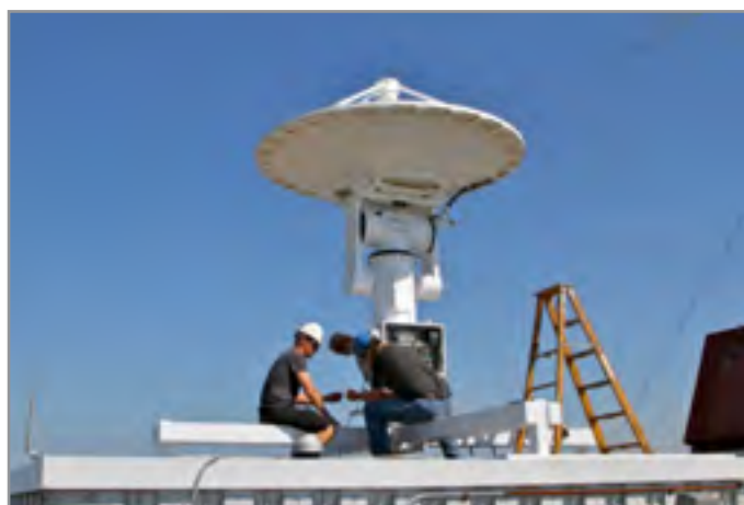
Figure 3. Installation of the SSEC X/L-band Direct Broadcast antenna on the UW-Madison campus in September 2011.
